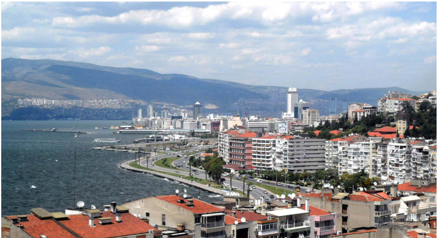
THE CITY OF IZMIR, TURKEY WAS DEVASTATED BY A MAGNITUDE SEVEN EARTHQUAKE ON OCT. 30, 2020. (PHOTO BY NEDIM ARDOĞA)
